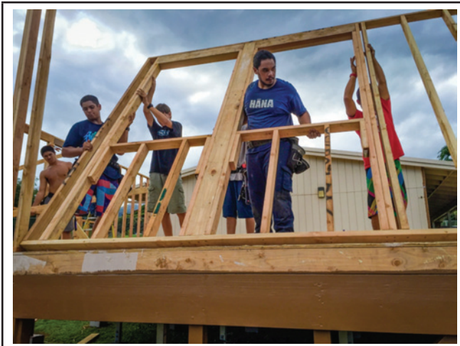
Figure 1. MKHKI Youth: Building a kupuna cottage as community caretakers.
